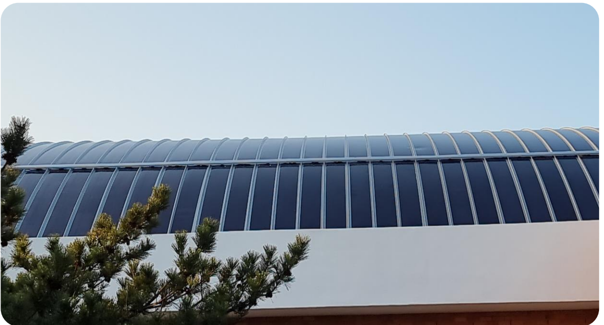
Roof of a gym_CIGS Flex 32Kw
