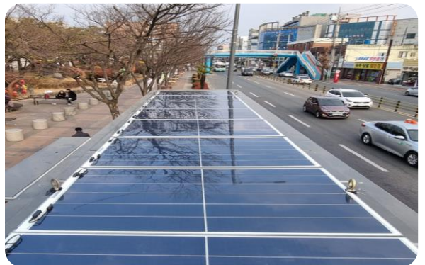
Jinju Bus stop_Mono Flex 9Kw
